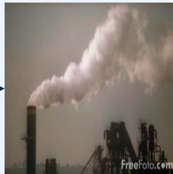
Electric Utilities And Suppliers
